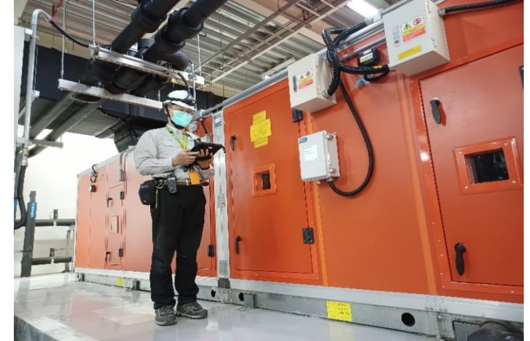
Air Handling Unit Equipment Maintenance
