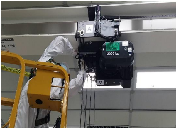
Cleanroom Overhead Crane Maintenance
